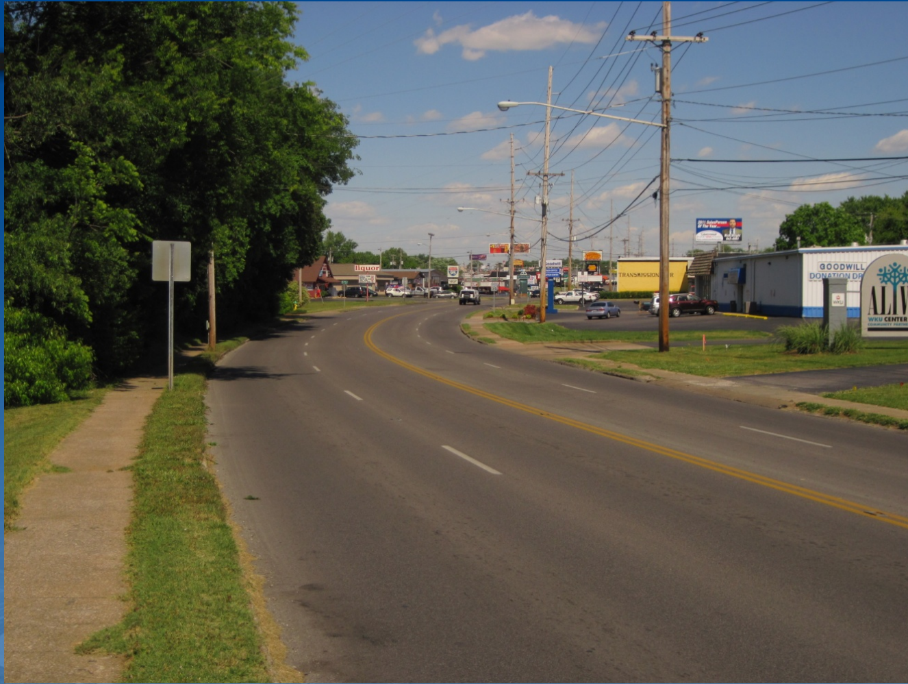
US 31W Bypass looking North, construction completed just after World War II.
